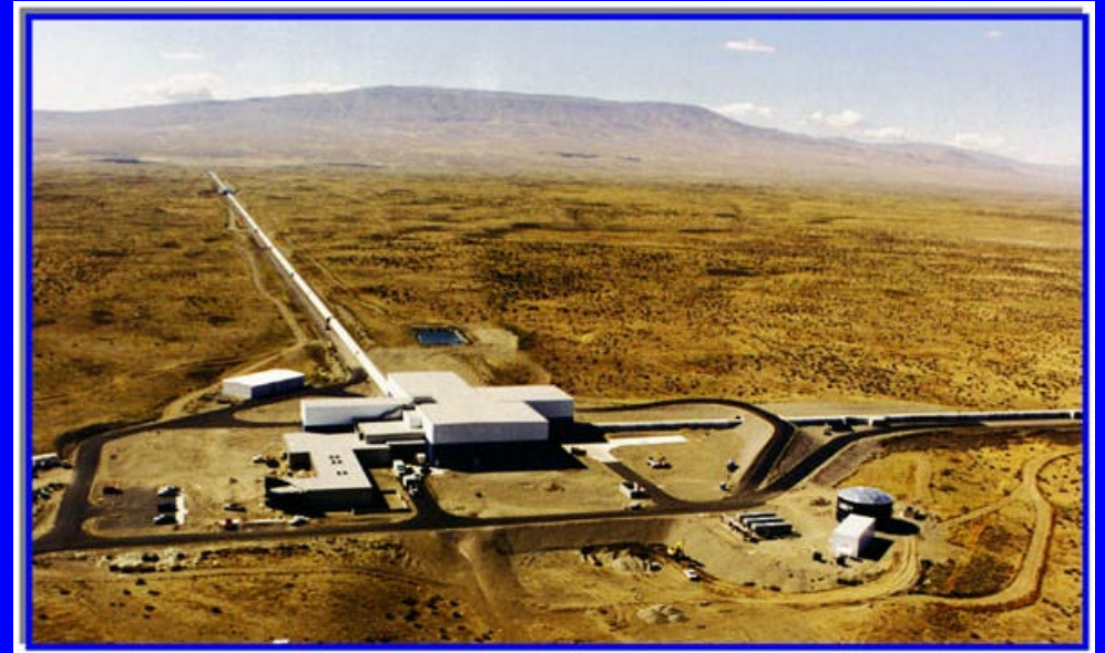
The Laser Interferometer Gravitational Wave Observatory (LIGO) installation near Hanford WA. Each interferometer arm is 4 km long. A similar instrument is located near Livingston LA ( www.ligo.caltech.edu )
